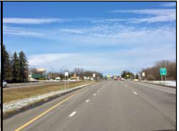
Hwy 169 Northbound View
