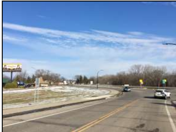
Hwy 99 Eastbound View
